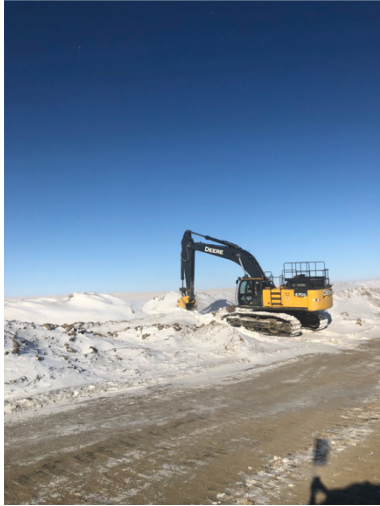
1. Excavator separating soil for Spring run-off – km 169+300 Feb 12, 2018
