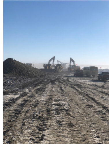
2. Clean up crew at wetland crossing – km 170+300 Feb 12, 2018
