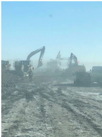
3. Clean up crew- km170+300 – Feb 12, 2018
